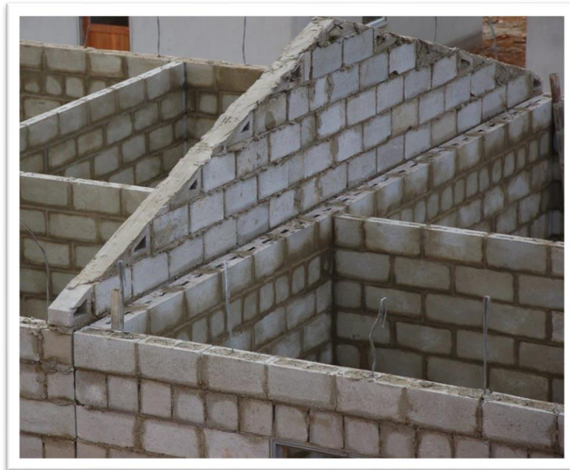
Figure 1 - Example of Modular Construction
